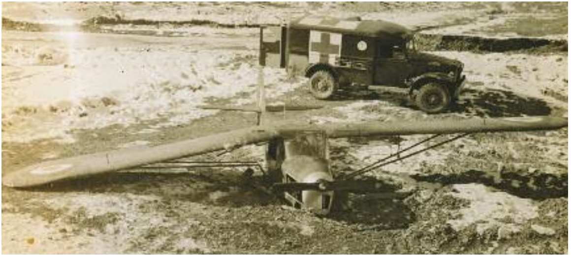
Auster fuel lines also froze in the Korean winters. This is TW425 having crashed on take-off on 4 December 1952. The pilot Capt Tees RCA, was unhurt.
